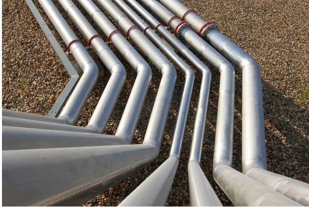
Connect the pipeline
